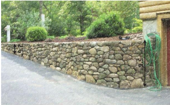
Figure 3-05. Retaining Wall Height
